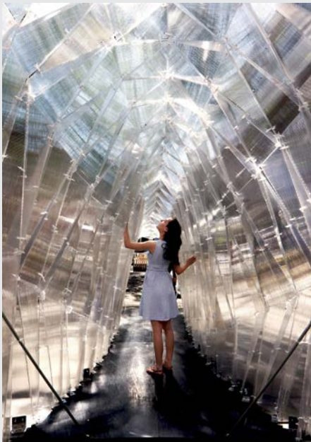
Created by 14 USC School of Architecture undergraduates, the "Glass Pavilion" installation was inspired by the simple form and folding techniques of origami designs. The structure had over 800 polycarbonate pieces fashioned into isosceles triangles, generating light reflections that provide unique spatial experiences. The students' blog about the installation generated interest as well as news stories.
